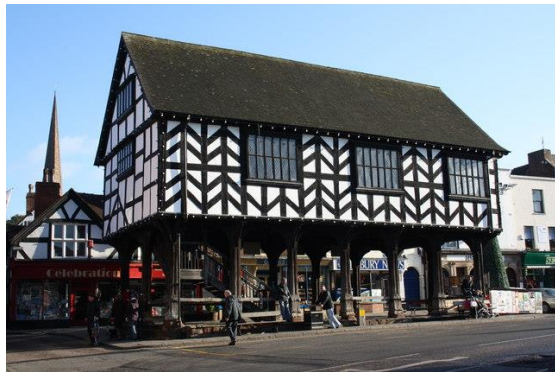
Figure 26: Ledbury Market House (Photo taken by David Cumberland)
