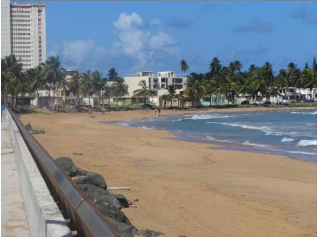
Figure 40: Beach and Concrete Wall at La Pared
