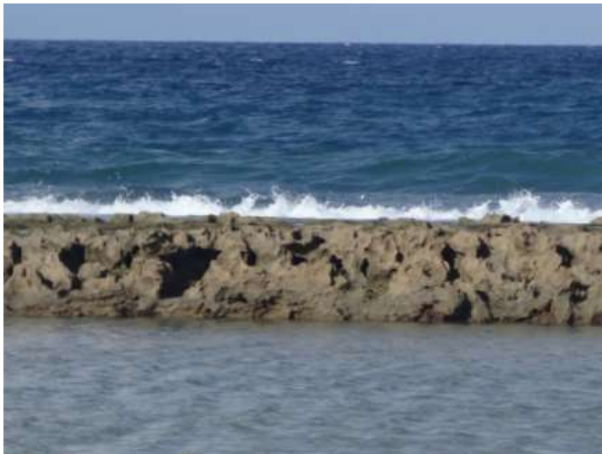
Figure 11: Wave Breaker at La Poceta
