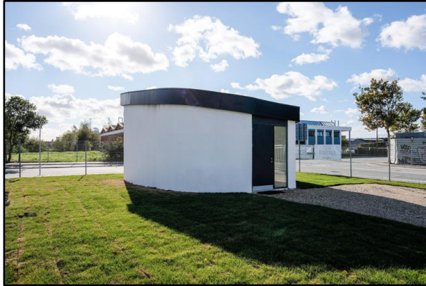
Figure 8: This image shows the finished product in Copenhagen (COBOD International, 2019).
