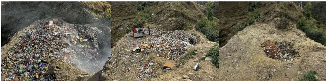
Figure 1515: Clearance progress of the waste dump (March 16, March 23, and March 28).
