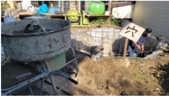
Figure 19: Concrete mixer and The Hole
