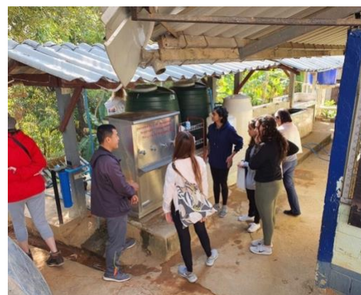
Figure 15. Learning about the water dispenser installed at Bamrung 87.
