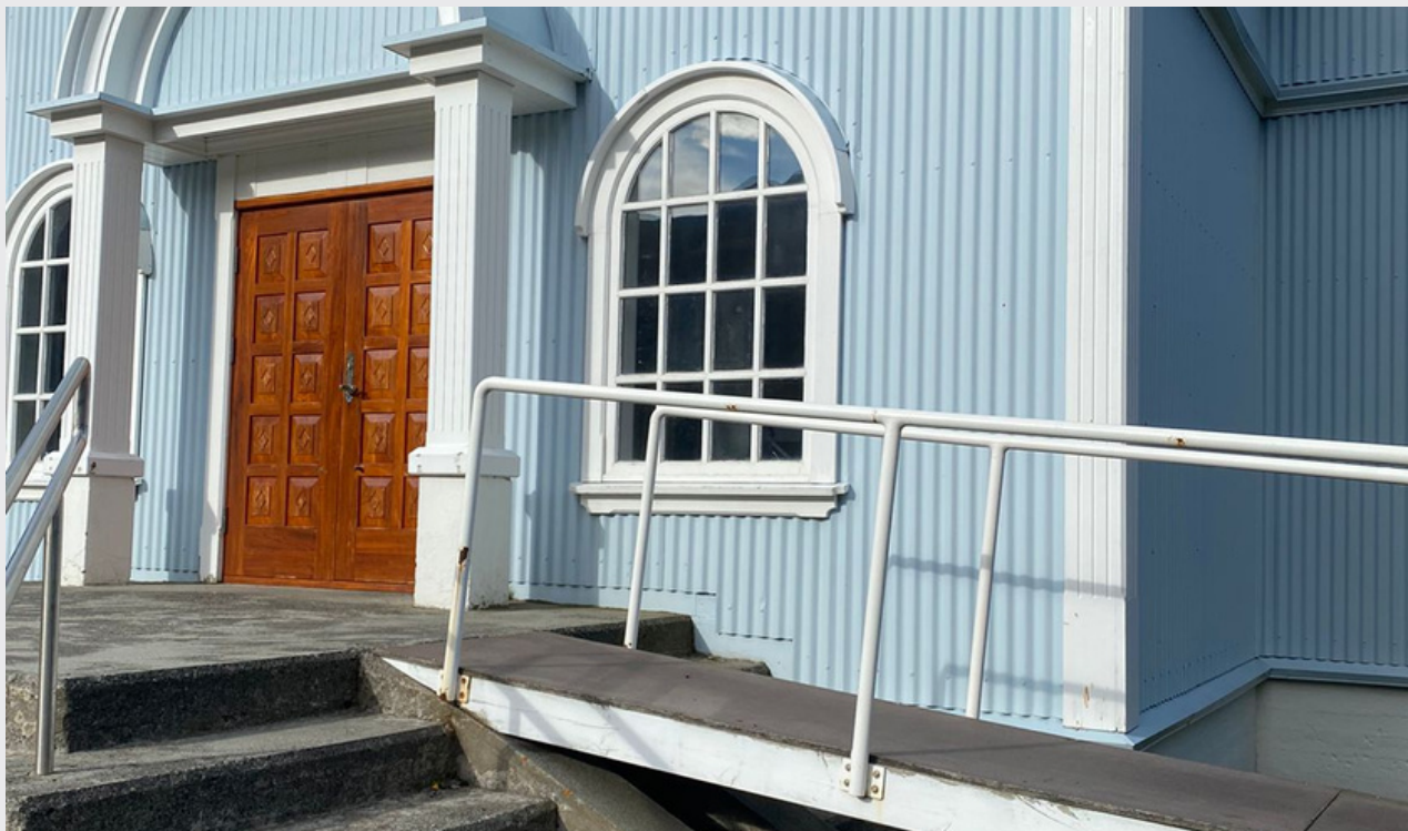
Figure 1. Image of ramp at a Lutheran church taken by Miguel Duran
