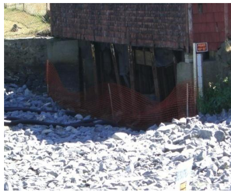
Figure 11. Current spillway condition showing gate house supports.
