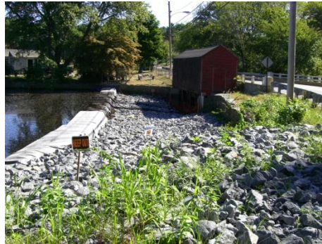
Figure 13. Temporary Cofferdam.
