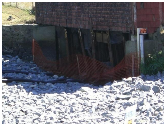
Figure 77. Spillway condition below the gatehouse.
