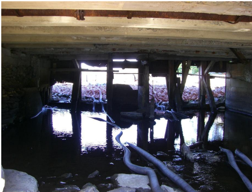
Figure 78. Downstream view of current spillway structure.
