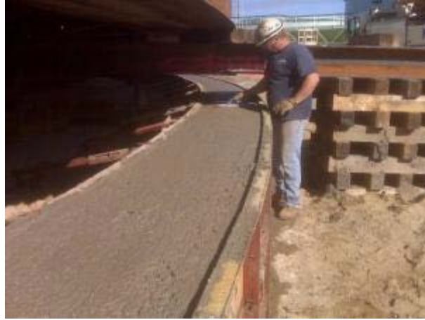
Figure 14: Concrete Finishing
