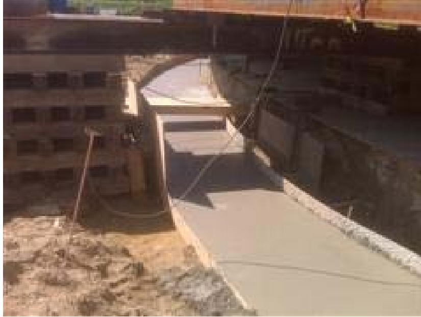
Figure 11: Concrete Footer Finish
