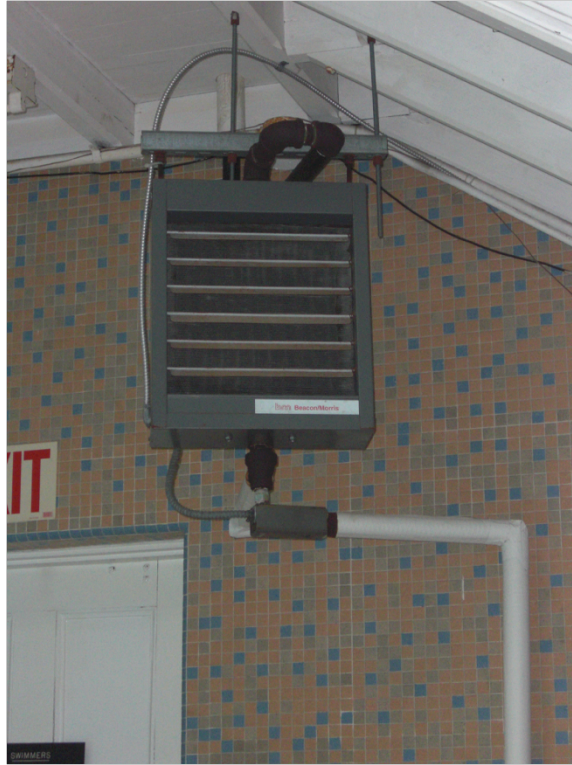
Figure 2-Steam Box Heaters
