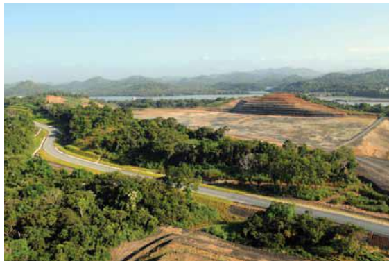
Figure 7: Relocation of the new Boriquen Road
