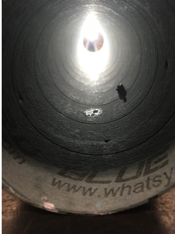
Figure 38. Actual placement of longitudinal strain gauge on the HPMR.
