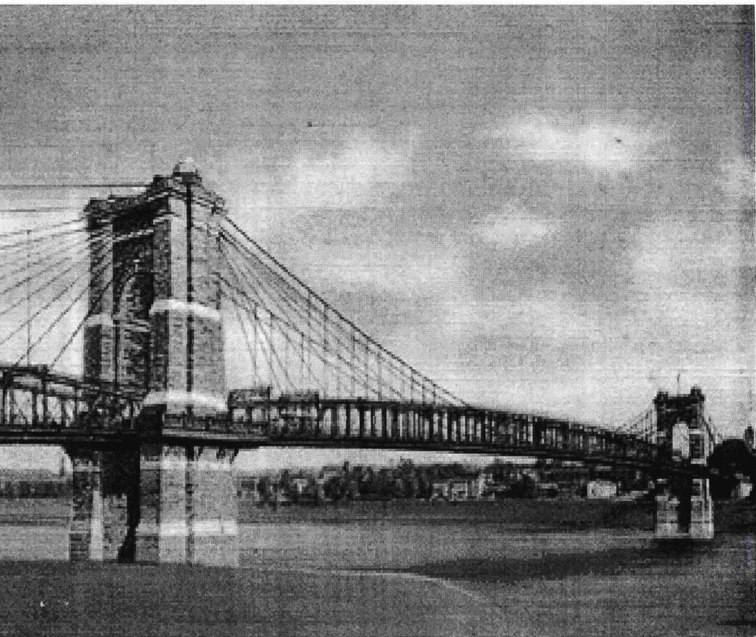
Roebling Suspension Bridge
