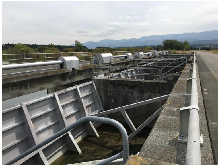
FIGURE 2.2 THE GEOFFREY BLUNDELL BARRAGE GATES
