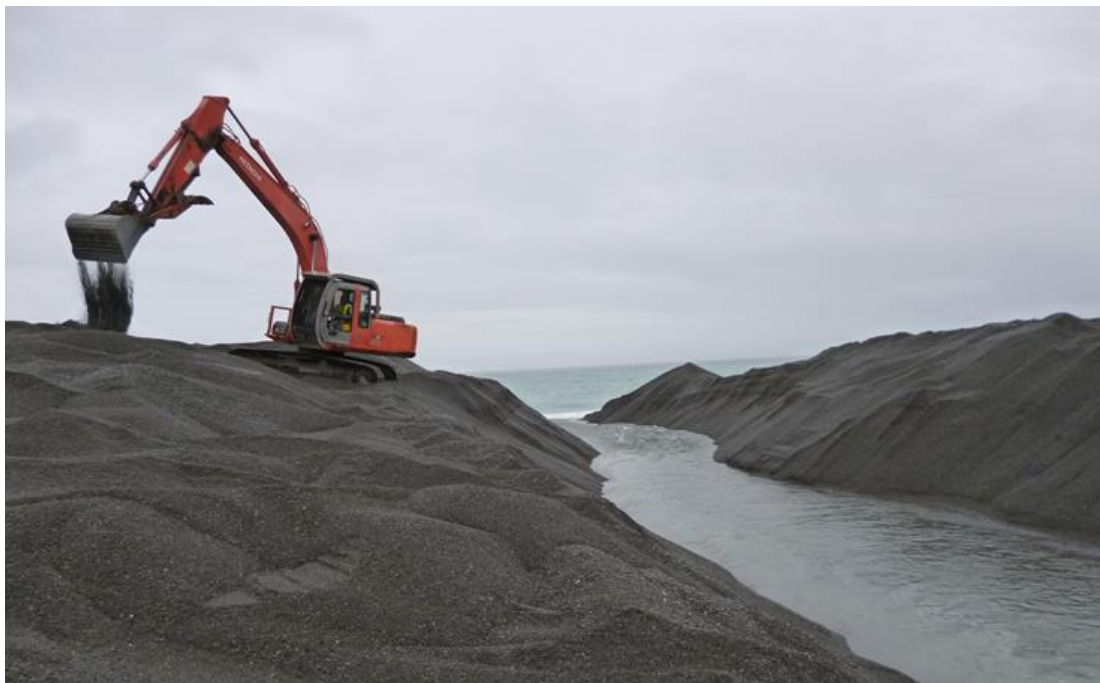
FIGURE 2.18 THE MECHANICAL OPENING OF THE LAKE ONOKE SPIT, [PHOTOGRAPH GWRC, 03/10/11]
