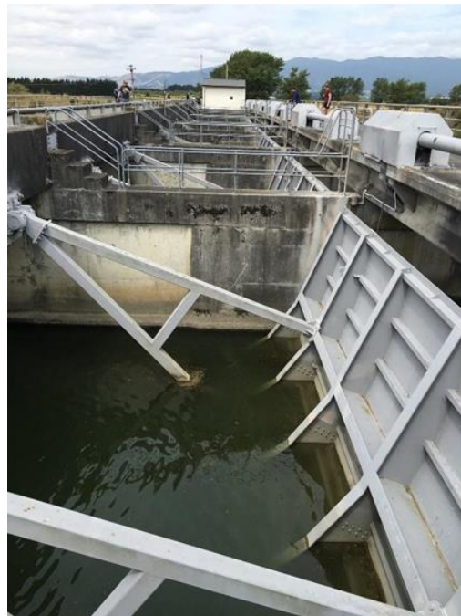
FIGURE 4.1 THE GEOFFREY BLUNDELL BARRAGE GATES
