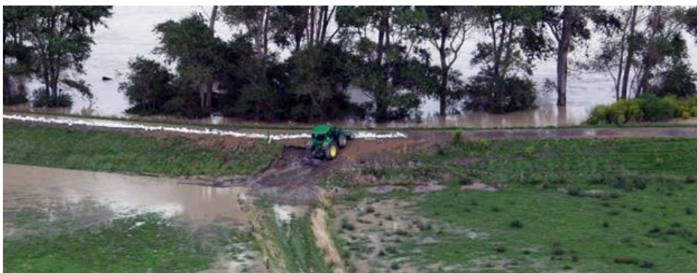
FIGURE 2.4 STOPBANKS ALONG THE RUAMAHANGA, [PHOTOGRAPH GWRC, N.D.]
