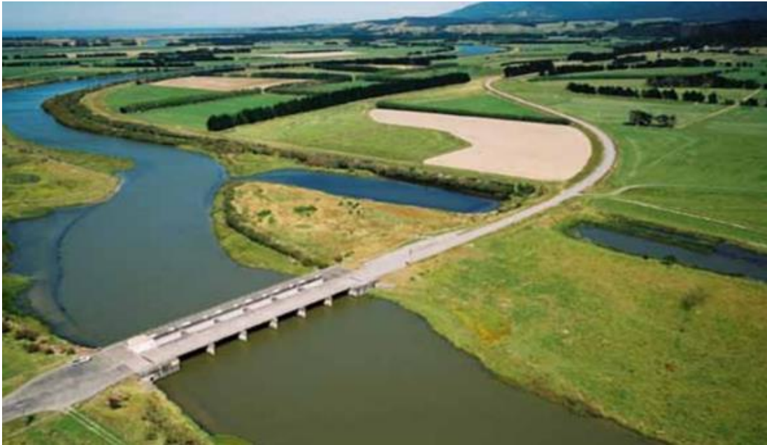
FIGURE 2.3 THE GEOFFREY BLUNDELL BARRAGE, [PHOTOGRAPH GWRC, N.D.]
