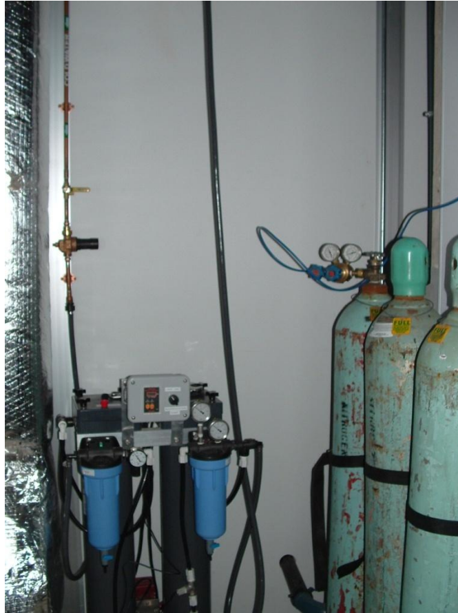
Figure D.1: Clean Room Supply Inlet
