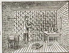
Registered Cellular Bins.
