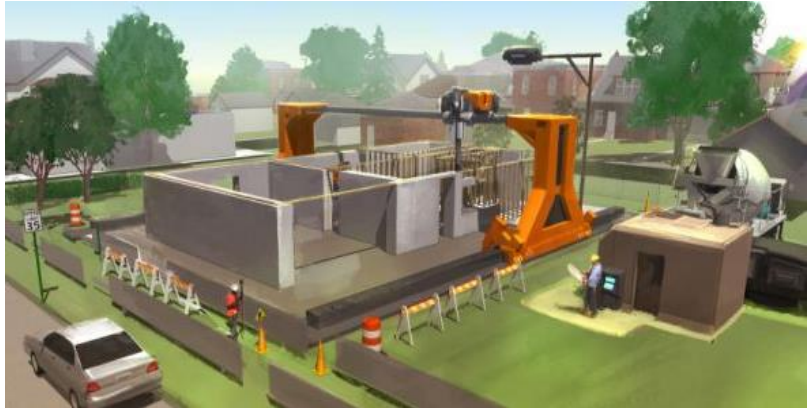
Figure 1: Automatic House 3D Printer
