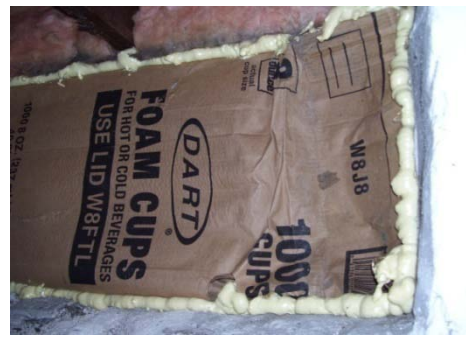
Figure 13: Properly Sealed Window
