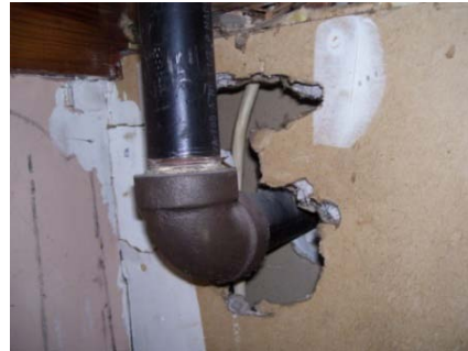
Figure 11: Unsealed Piping
