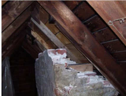
Figure 10: Open Chimney in
