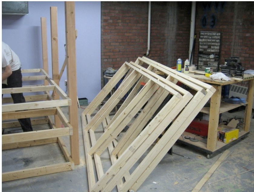
Dom works hard as the flat wood storage starts to come together.
