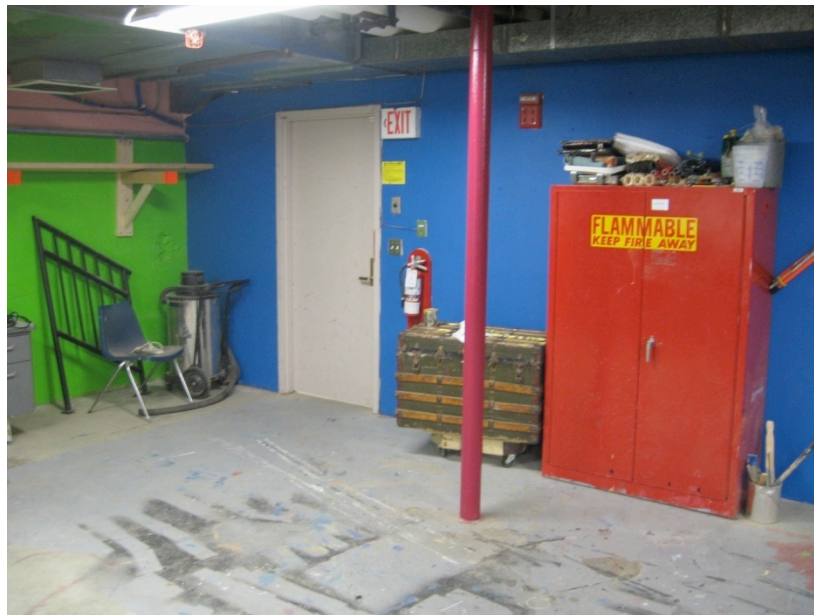
The fire escape is now accessible.
