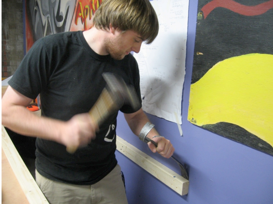
Chris removes a 2x3 from the wall.
