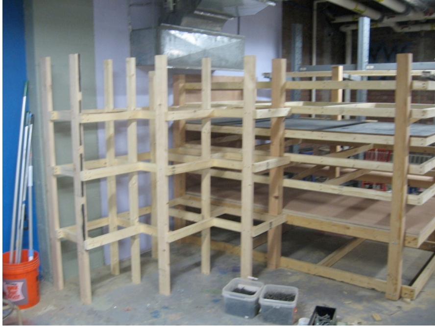
The completed flat wood storage, and cut lumber storage areas.
