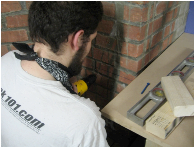
Dom mounts wood directly into the brick using masonry screws.
