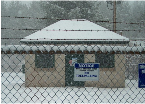
Figure 9- Lee Street Pump Station
