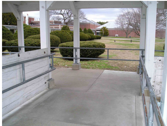
Figure 4: Outdoor walkway (pergola) at MHS lined with metal railings
