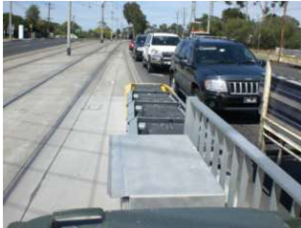
Figure 15: Stop 65 - Compressive Barrier
