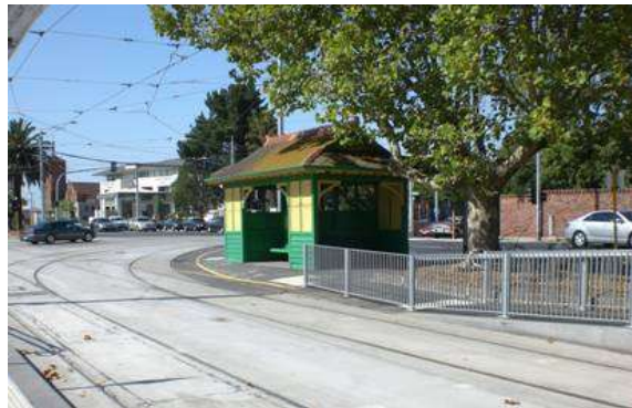
Figure 19: Stop 48 - Heritage Building and Intersection
