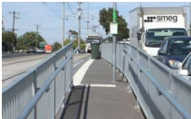
Figure 16: Stop 65 - Narrowing Stop Width
