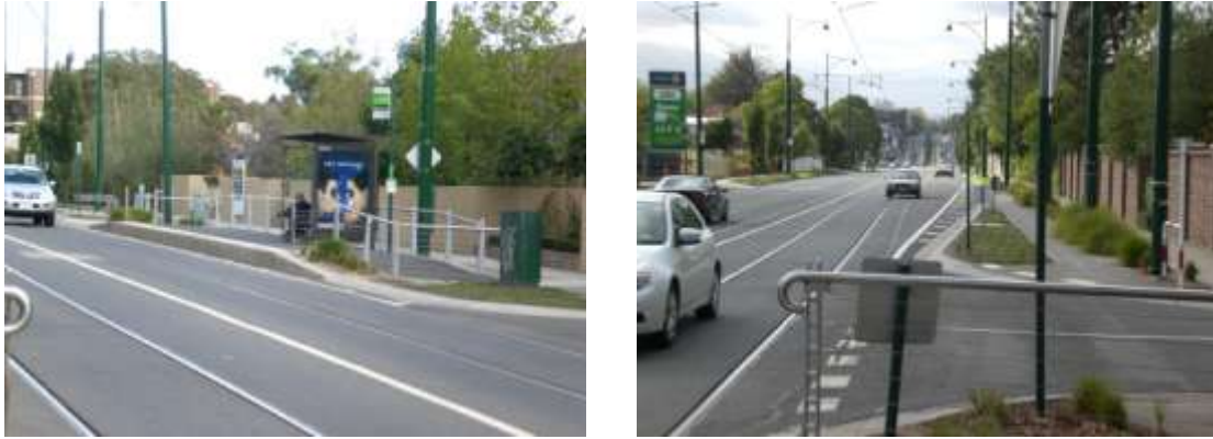
Figure 22: Kerb Access Stop
