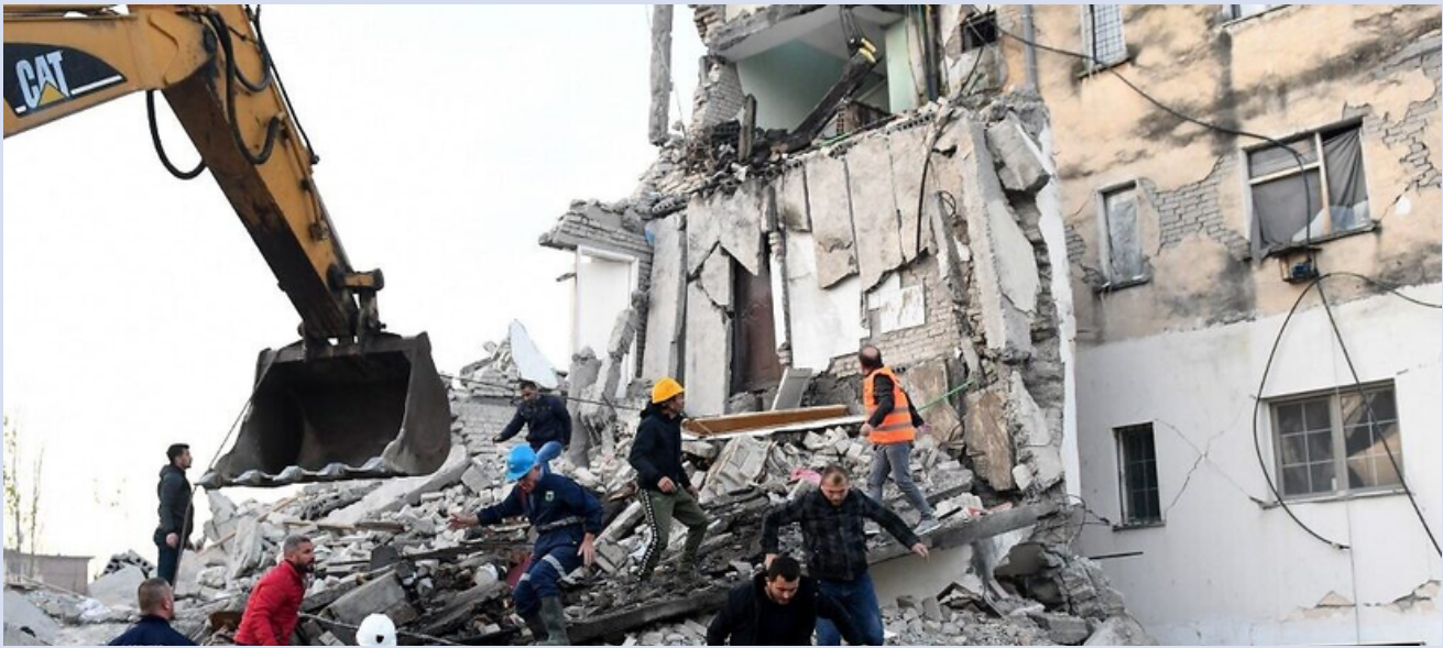
Figure 6. Damages from the 2019 Earthquake
