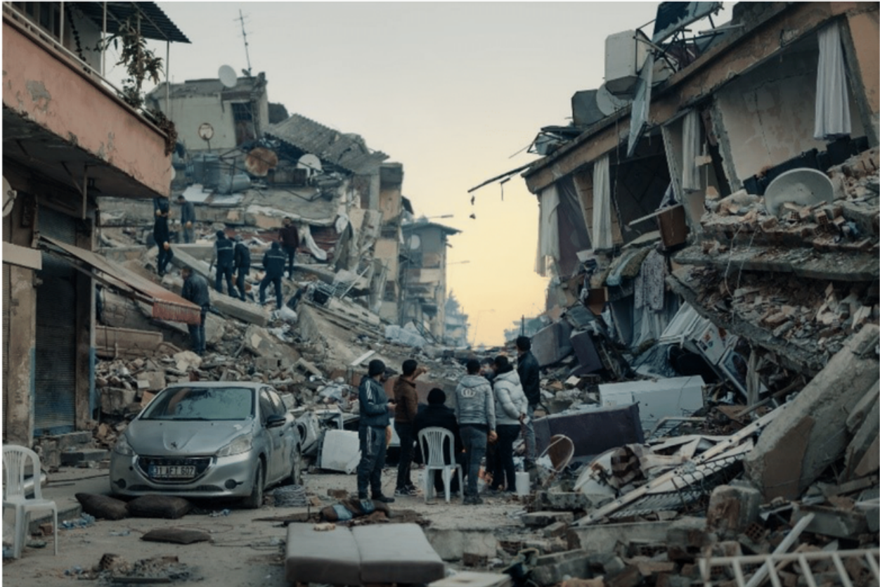
Figure 1: Damage in Ankara, Turkey (NY Times, 2023)
