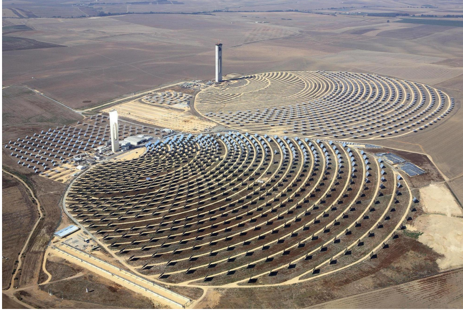
Figure 10: Solar power plant (Papundits World Press).
