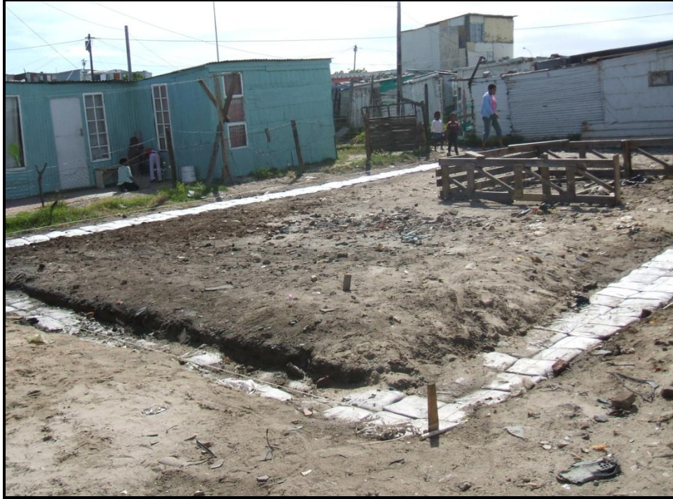
Figure 4.6: Indlovu Sandbag Community Centre Foundation
