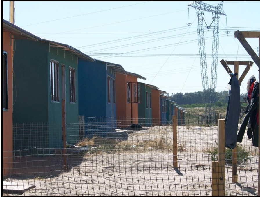
Figure 4.7: Witsand iEEco Houses Shaded by Roof Overhang in Summer
