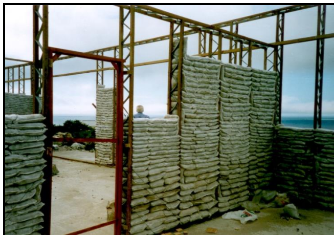
Figure 2.10: Eco-beam Technology Being Used to Build a House
