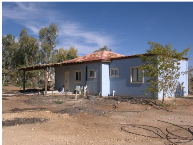
Figure 4: Northwest facing side of Iris' house
