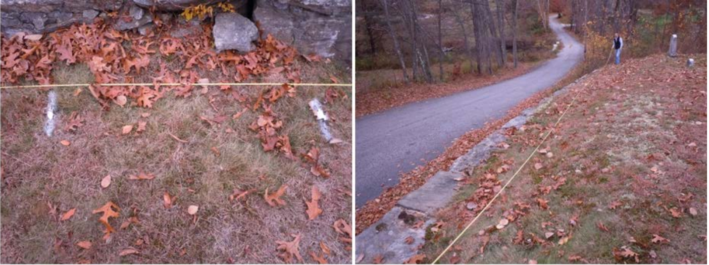
Figure 8: Use the measuring tape and spray paint to mark the gridlines
