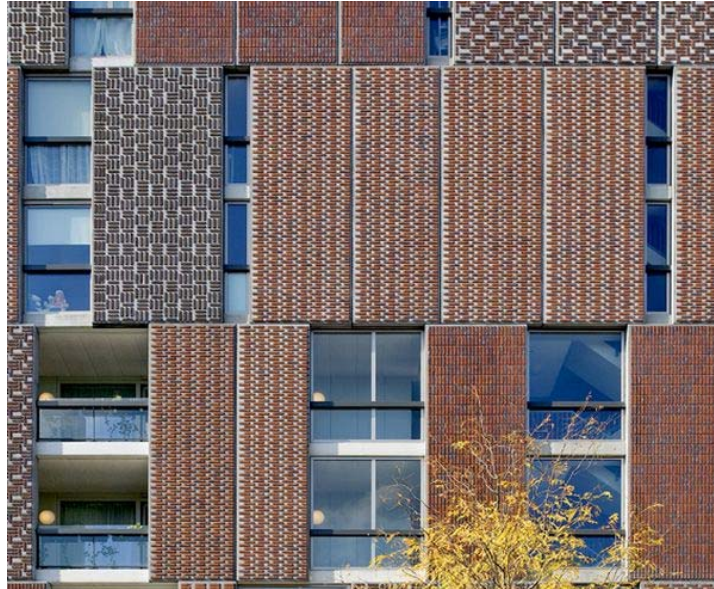
Figure 11: Precast Panels with Brick Inspiration
