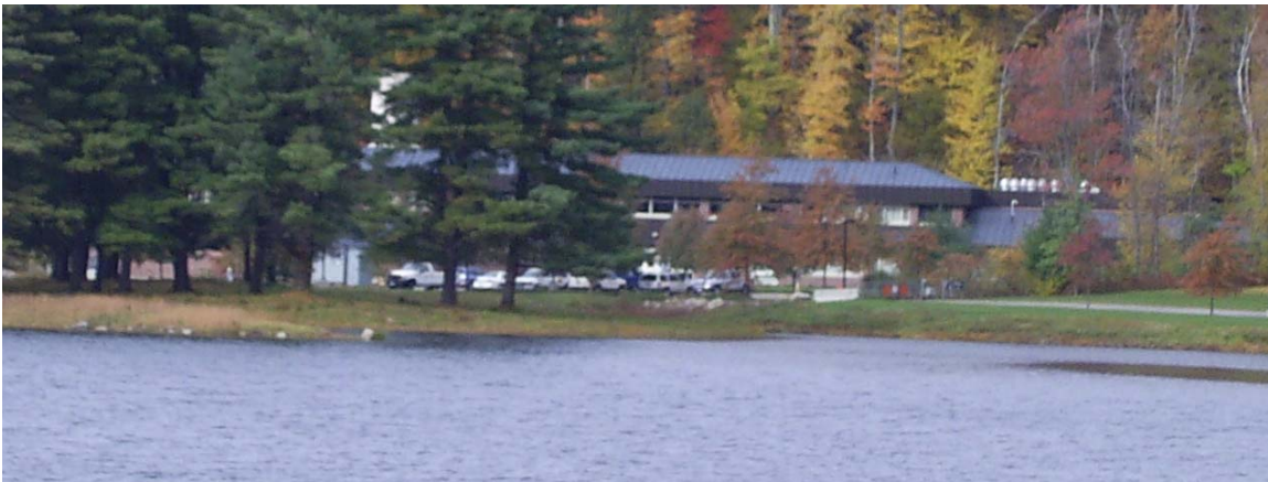
Figure 9. The Worcester DPW Treatment Facility in Holden, Massachusetts
