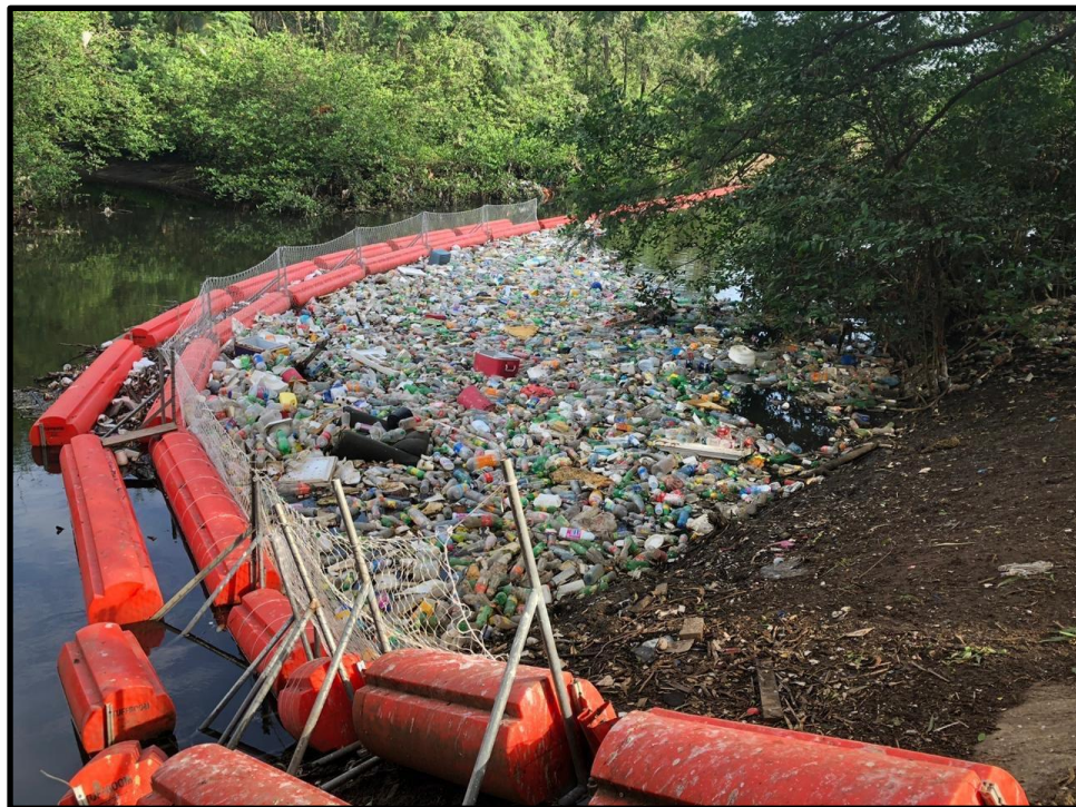
Figure 2-3: Marea Verde’s “Barrera o Basura” trapping waste on the Matías Hernández River (Marea Verde, 2018).
