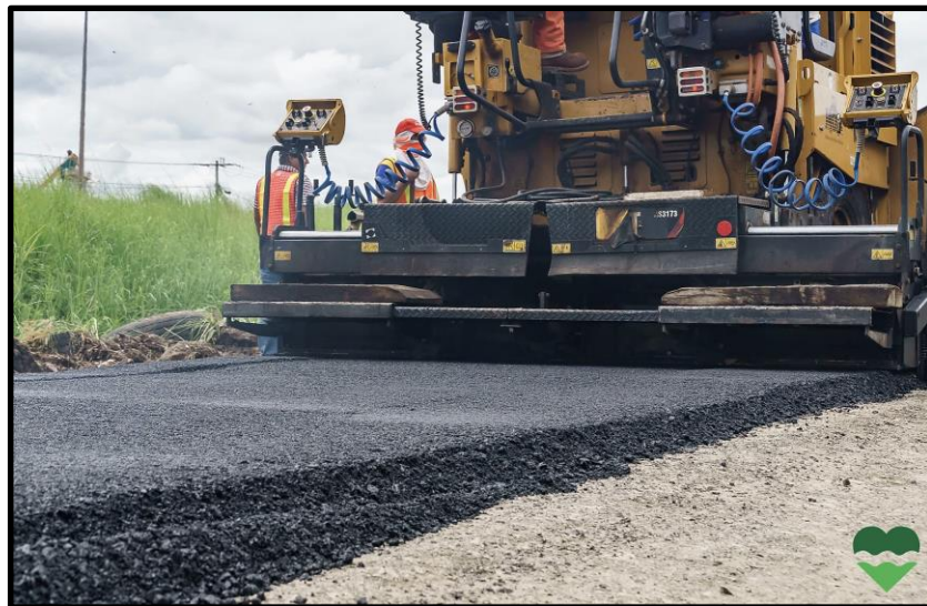
Figure 2-4: The first pilot project for paving roads (Marea Verde, 2018).
