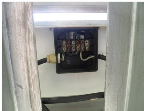
FIGURE 28: EXPOSED WIRES
