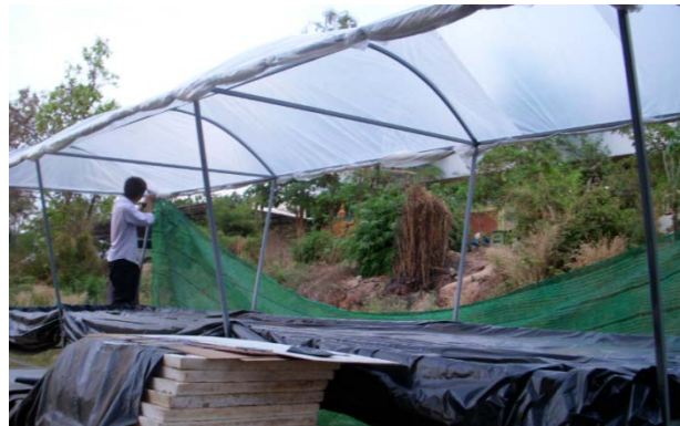
Figure 1: The Semi-Quonset Design (Left) Figure 2: Constructed Hydroponic System (Right)
