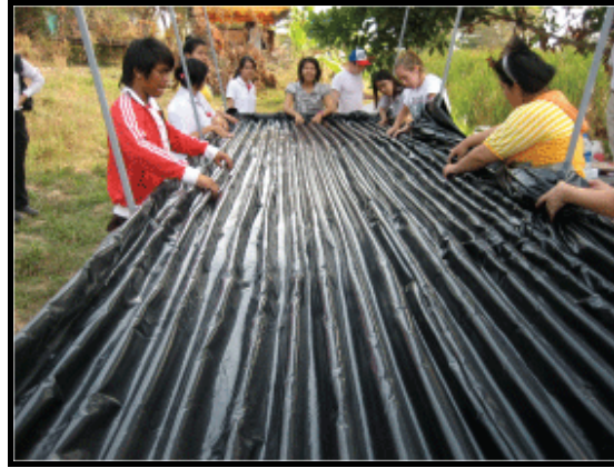
Figure 21: Construction of the System
