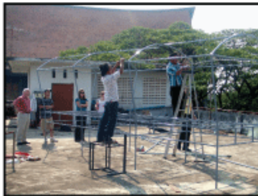
Figure 20: Fabrication of the Frame
