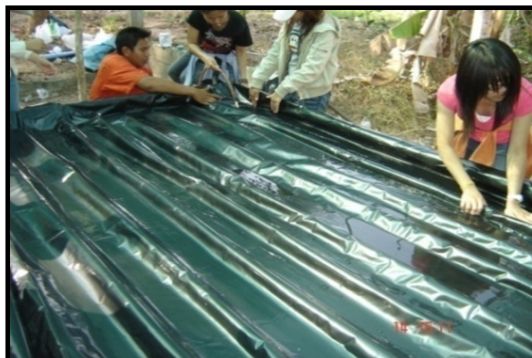
Figure 12: Lining of the Channels with Polyethylene Plastic in the MSU SIFE Team Hydroponic System (Left) Figure 13: Plastic Sheeting for Roof and Mosquito Nets on the Sides in the MSU SIFE Team Hydroponic System (Right) Source: Kid-Arn (2008)
