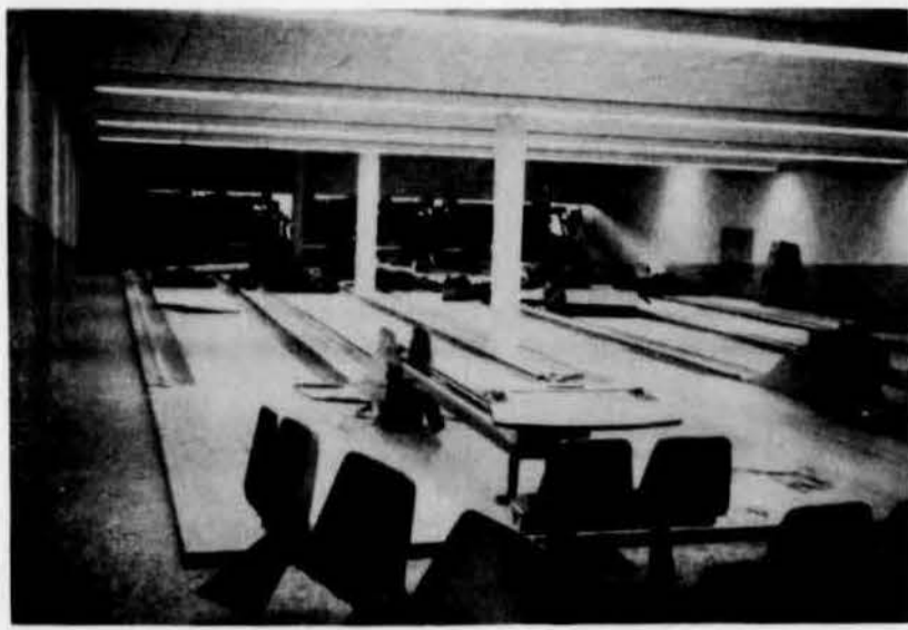
New Lanes Near Completion
