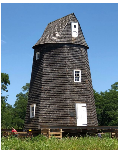
Figure 2.3.2: Raising of the Foundation (Shelter Island Reporter, 2018)
