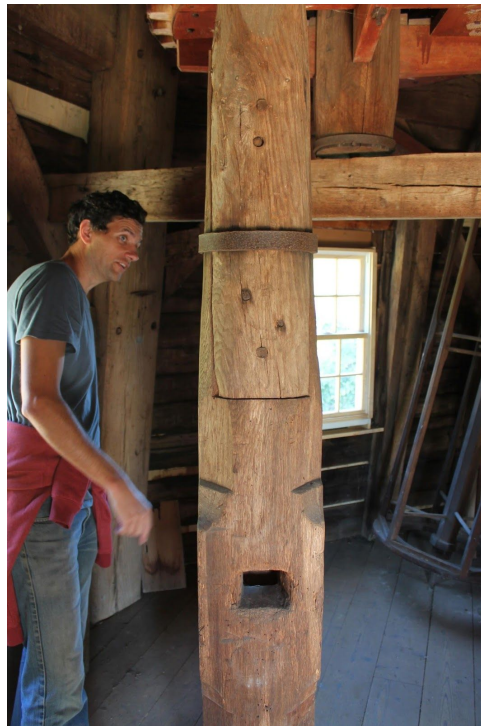
Figure 2.3.3: First Floor Turret (Campbell, 2019)
