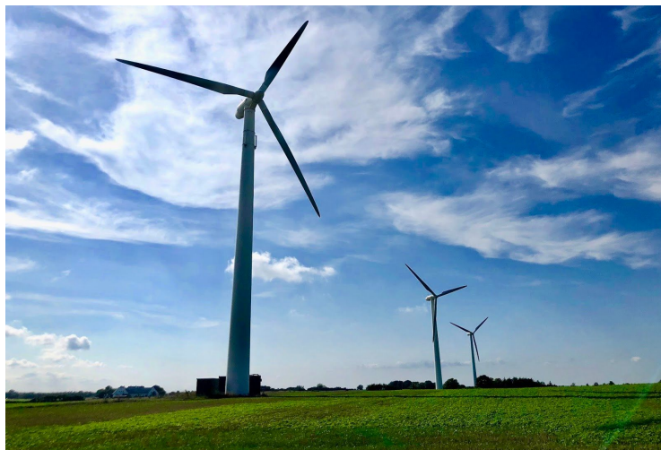
Figure 2.4.1: Modern Wind Turbines (Campbell, 2018)
