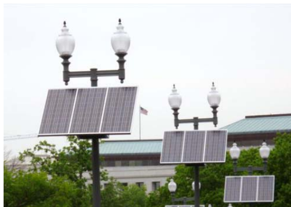
Figure 2-4: Solar Street Lights by Sol Inc. (Palm City, FL)
