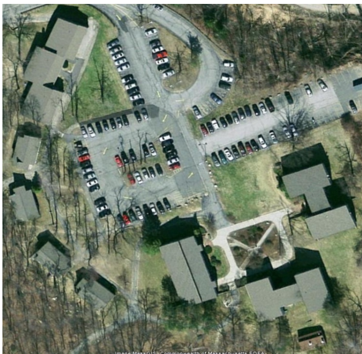
Figure 2-6: Aerial View of Assumption College Dormitories (Source: Google Earth)
