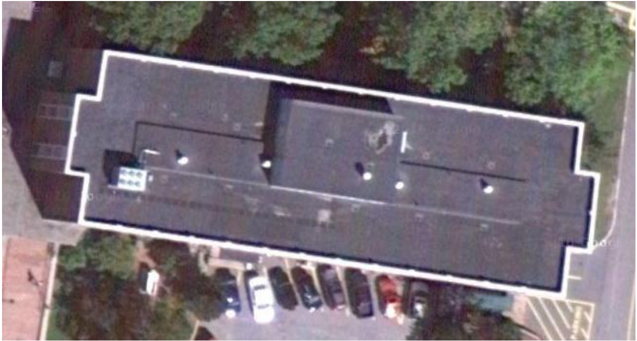
Figure 18: Daniels Hall Roof Top [15]
