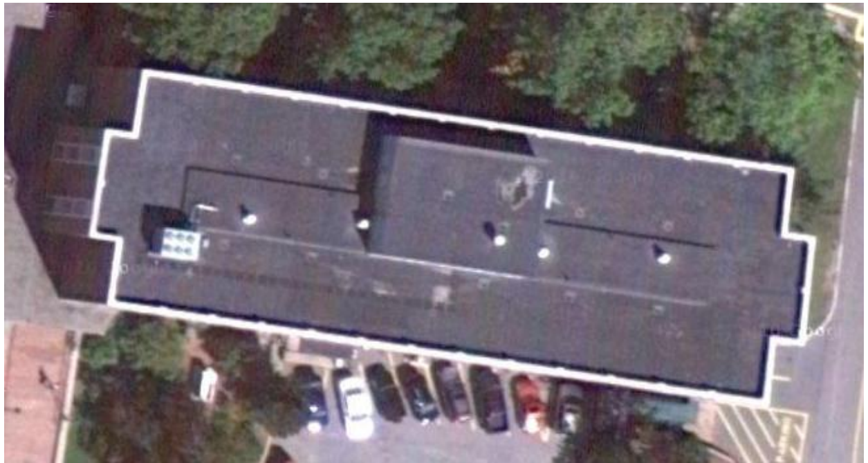
Figure 12: Google earth image of Daniels Hall rooftop [15]
