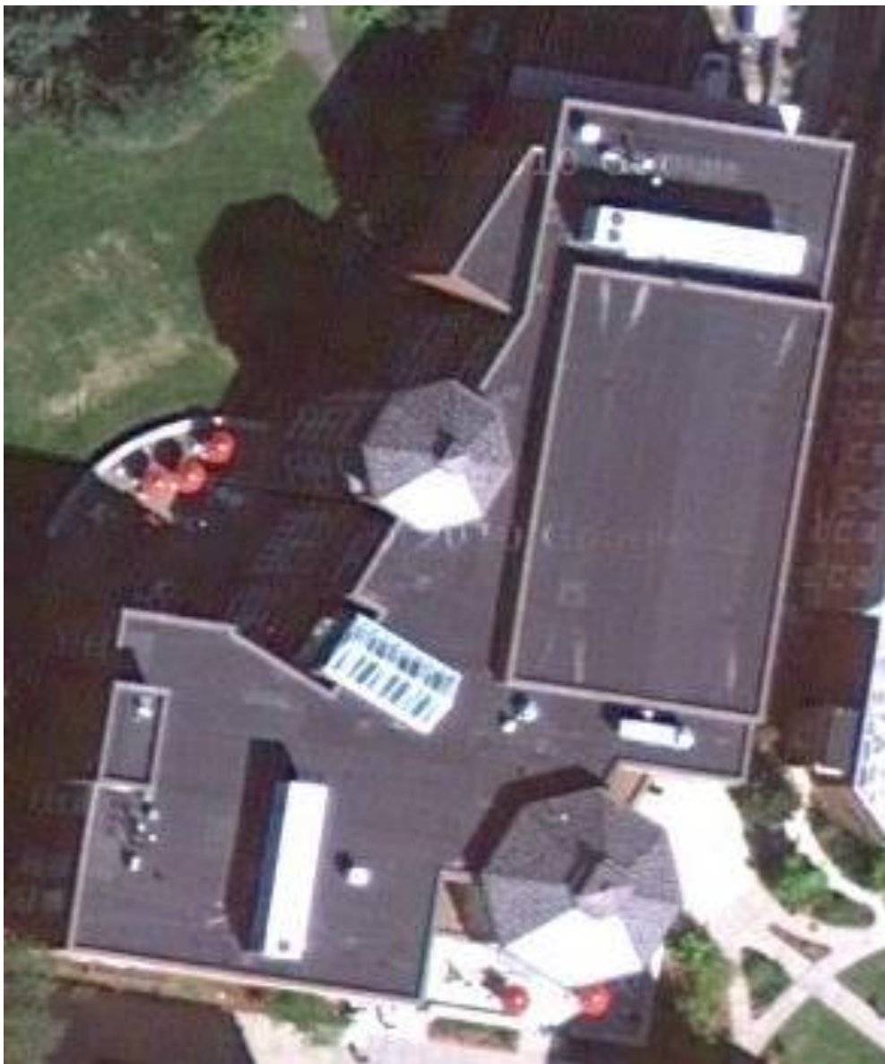
Figure 13: Google Earth image of Campus Center rooftop [15]
