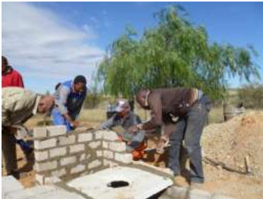
FIGURE 50: (LEFT) TOILET HOUSE WALLS BEING BUILT
