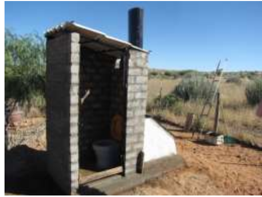
FIGURE 51: (RIGHT) CONSTRUCTION OF TOILET HOUSE WALLS CONTINUES
