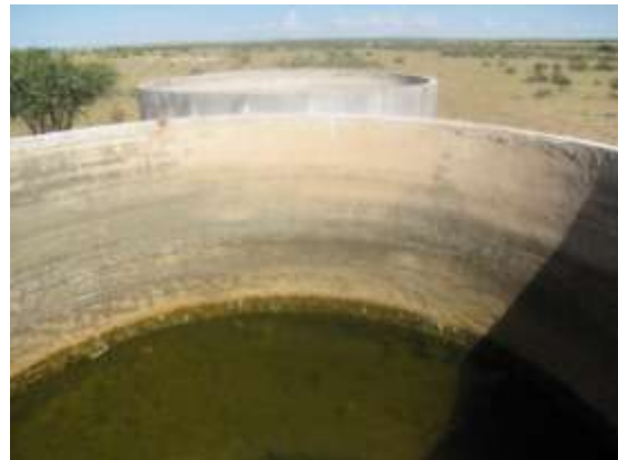
FIGURE 32: (RIGHT) SEVERE BIOLOGICAL GROWTH IN THE EXPOSED RESERVOIRS
