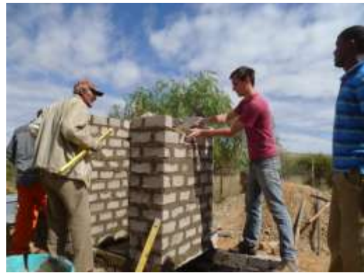
FIGURE 51: (RIGHT) CONSTRUCTION OF TOILET HOUSE WALLS CONTINUES
