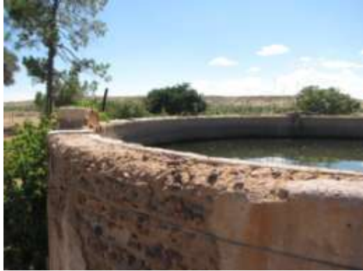
FIGURE 19 A AND B: EDGES OF THE RESEVOIR SHOW SIGNS OF CRACKING AND PIPES ARE RUSTING
