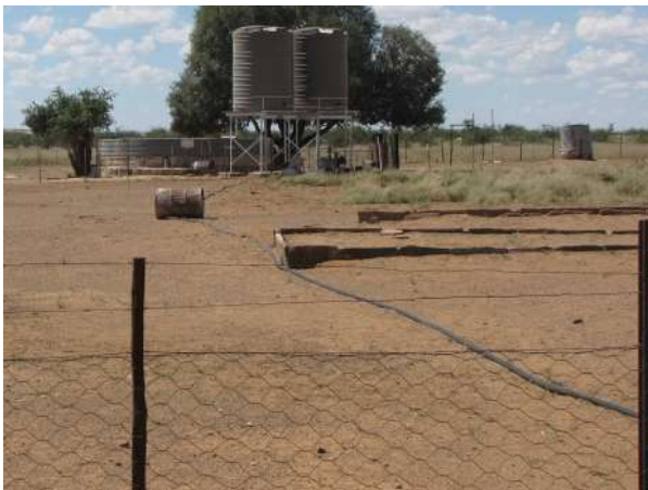
FIGURE 17: (LEFT) RUBBER PIPING ABOVE GROUND, ALTHOUGH APPEARS IN GOOD CONDITION
