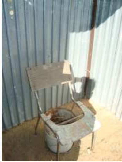
FIGURE 3: THE BUCKET SYSTEM
