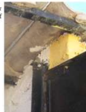
south door roof
