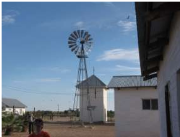
FIGURE 22: (LEFT) WINDMILL POWERED BOREHOLE IN CENTER OF COMMUNITY
