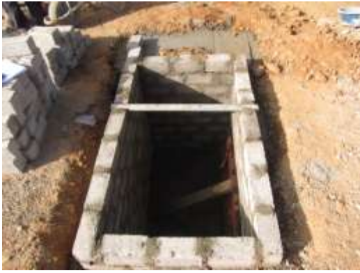
FIGURE 48: (LEFT) MR. GEORGE ADDED A HORIZONTAL SUPPORT INTO THE DESIGN
