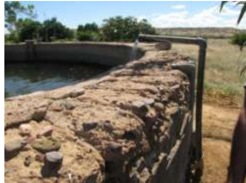
FIGURE 19 A AND B: EDGES OF THE RESEVOIR SHOW SIGNS OF CRACKING AND PIPES ARE RUSTING
