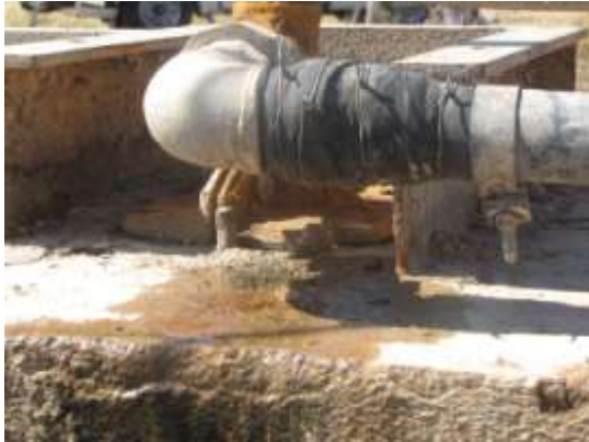
FIGURE 30A AND 30B: TEMPORARY SOLUTIONS TO LEAKY PIPES
