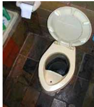
FIGURE 56A AND B: UDS COMPLETE CONSTRUCTION DESIGN AND URINE DIVERSION SYSTEM (WIENECKE 2011)
