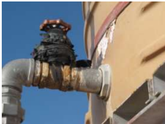
FIGURE 24: (LEFT) A LEAKING PIPE FROM A STORAGE TANK IS PATCHED
