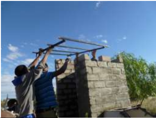
FIGURE 52: (LEFT) ROOF SUPPORT IS ADDED
