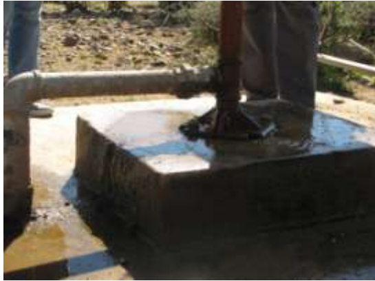
FIGURE 12: (LEFT) BOREHOLE BASE SHOWS SIGNS OF RUSTING AND LEAKING
