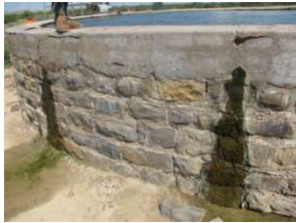
FIGURE 34: (RIGHT) BIOLOGICAL GROWTH ALONG THE LEAKS IN THE DAM
