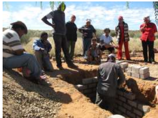
FIGURE 46: (LEFT) MR. GEORGE AND THE LOCAL MASON LAY BRICKS
