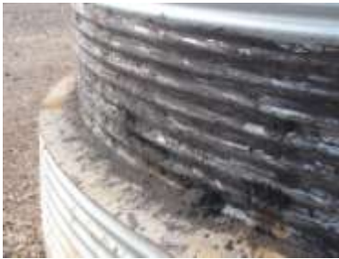
FIGURE 27A AND 27B: SUCCESSFUL REPAIRS TO THE SECOND RESERVOIR
