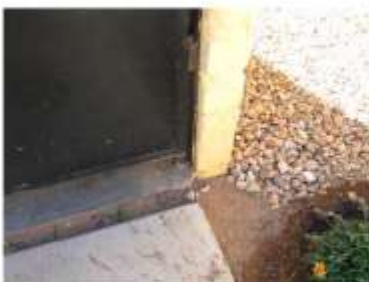
south door floor
