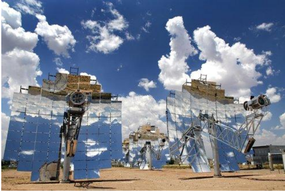
Dish-engine solar system. The solar dish generates electricity by focusing the sun's rays onto a receiver, which transmits the heat energy to a Stirling engine, which in turn drives a generator to make electricity. (Sandia National Laboratory) 3
