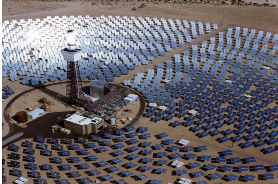
Stretched membrane heliostats with silvered polymer reflectors will be used as demonstration units at the Solar Two central receiver in Daggett, CA. (Sandia National Laboratory) 32
