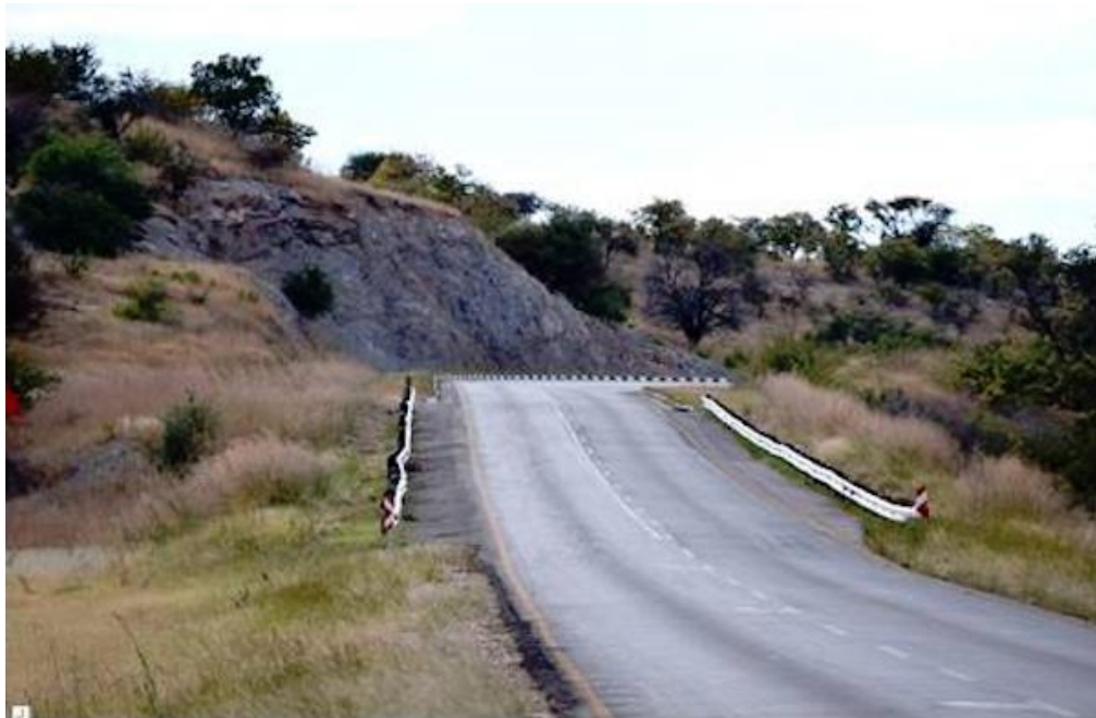
Figure 48. Blind Spot due to a Curve on Stretch 85 on B1
