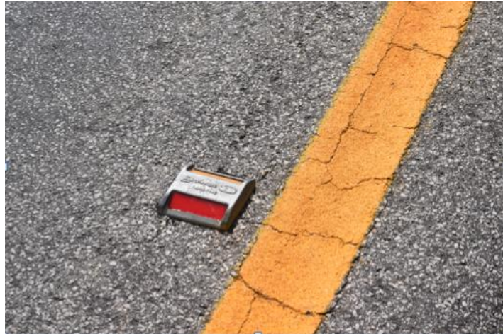
Figure 61. Reflective road tag on Stretch 85 on B1
