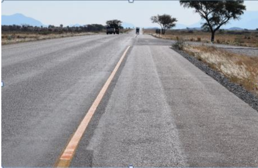
Figure 63. Expanded Roadway on Stretch 9
