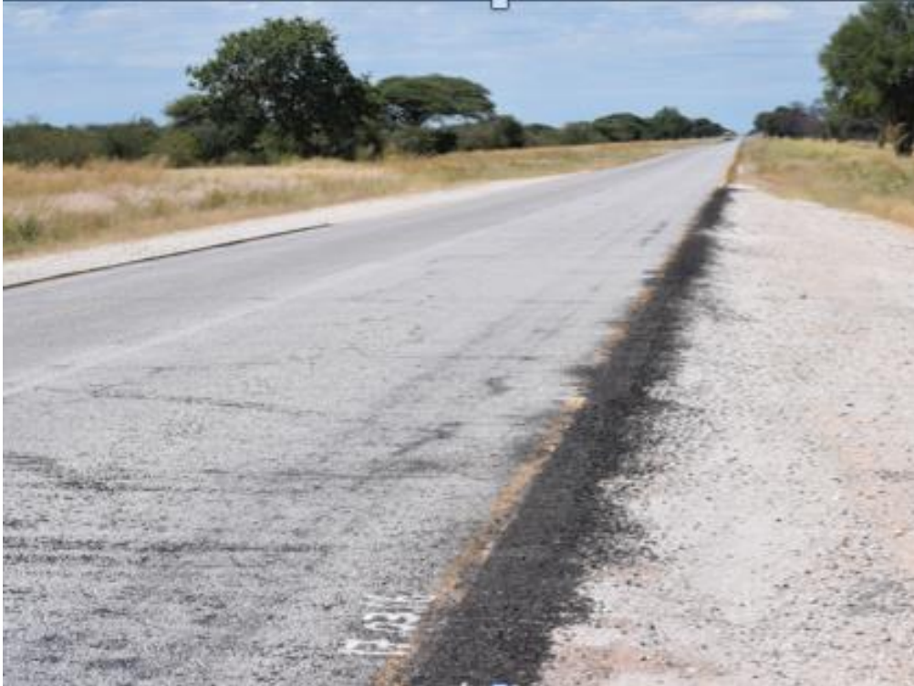
Figure 64. A Paved Drop-off on Stretch 94
