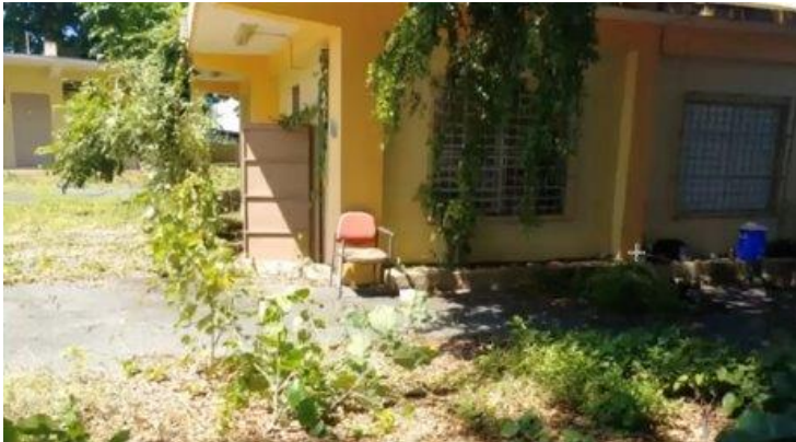
Figure 23: Sociedad Sembry Planet's vacant facilities before proper maintenance was completed.
