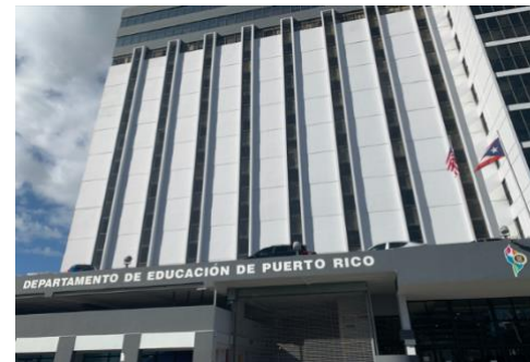
Figure 5: The department of education headquarters in San Juan, Puerto Rico.
