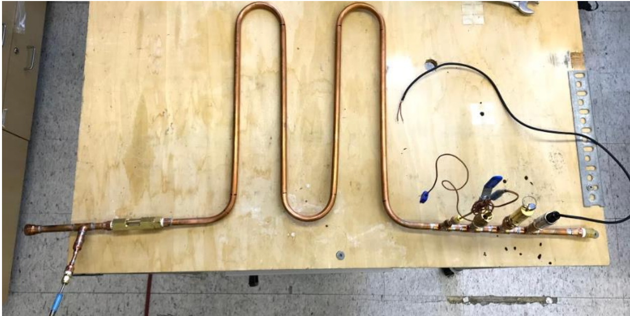
Figure 21: Condenser with instruments added
