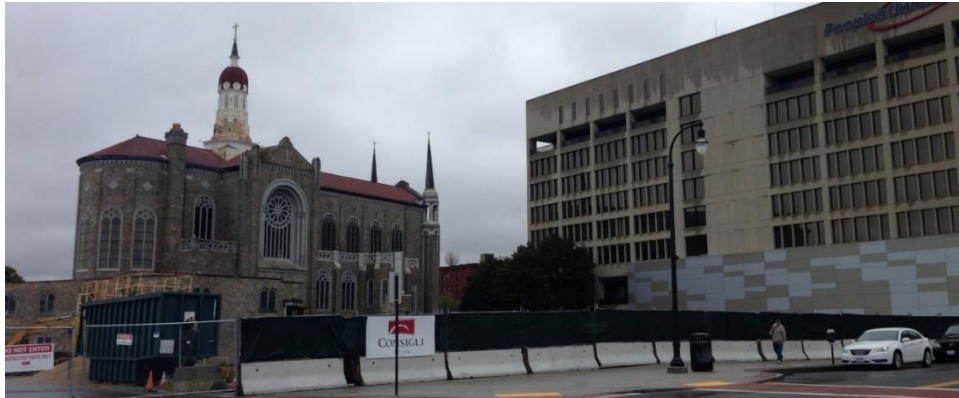
Underground Parking Garage Site from Front St. View
