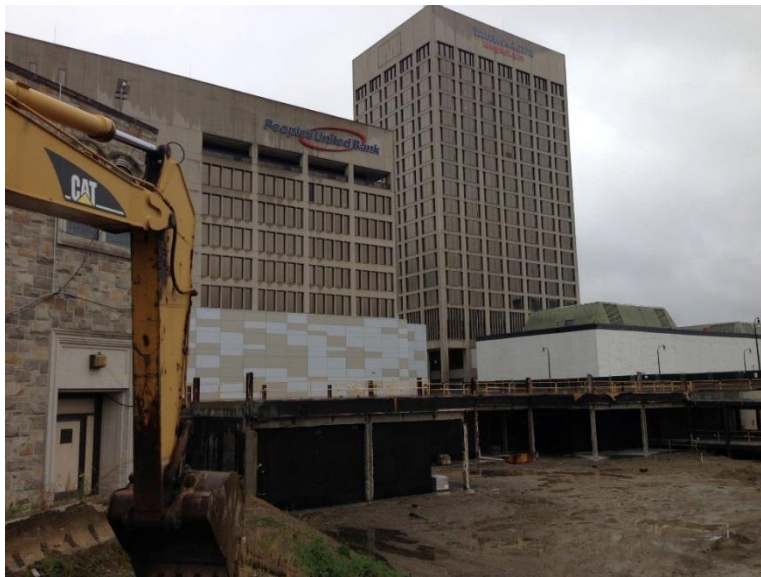
Building E Area from Trumble St. View
