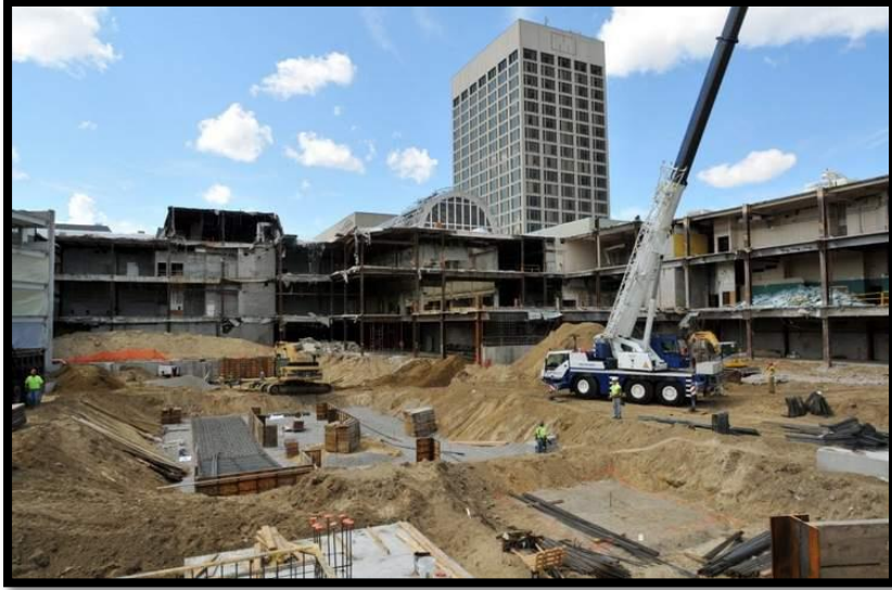
Figure 5 - Demolition of Worcester Commons Fashion Outlets (Grillo, 2013)
