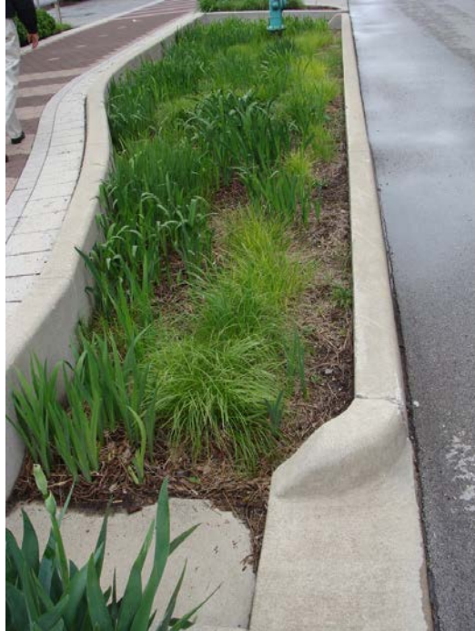
Figure 6: A bioswale next to a road (National Association of City Transportation Officials, 2016).
