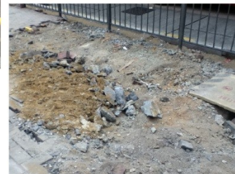
Figure 1: Two different main types of construction and demolition waste: non-inert waste, such as bamboo and cardboard, and inert waste, such as brick, metals, and rocks.
