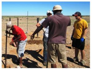
Figure 13. Hole digging using a heavy handle to separate the sand from the gravel
