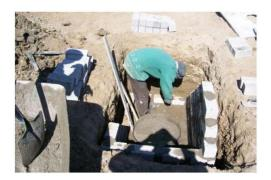
The walls of the underground tank can be build out of super bricks or any other bricks which are available. Just make sure that you keep the inside measurements shown in the construction plan. The walls must reach one brick over ground level.
