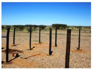
Figure 14. Support poles in cement left to set in the sun
