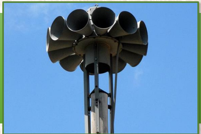
Figure 10: Tornado siren in Boulder with wildfire alert capabilities (photo credit: “Emergency Warning Sirens,” n.d.).
