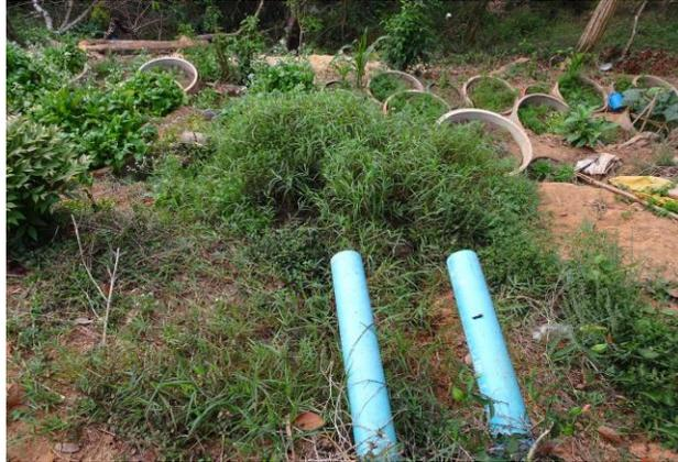
**Figure 9: Pipes draining over Terrace Garden**
