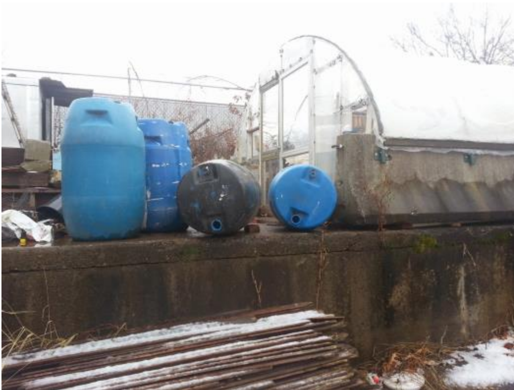
Figure 10: Location of the digester before construction.
