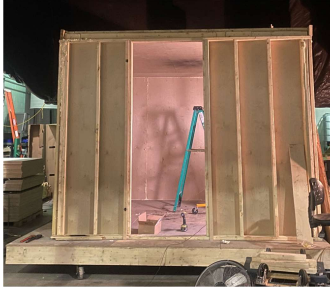
Figure 8: Picture of reduced -scale enclosure during construction.
