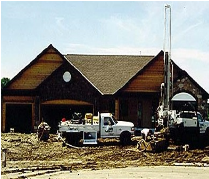
Installation of the geothermal system
